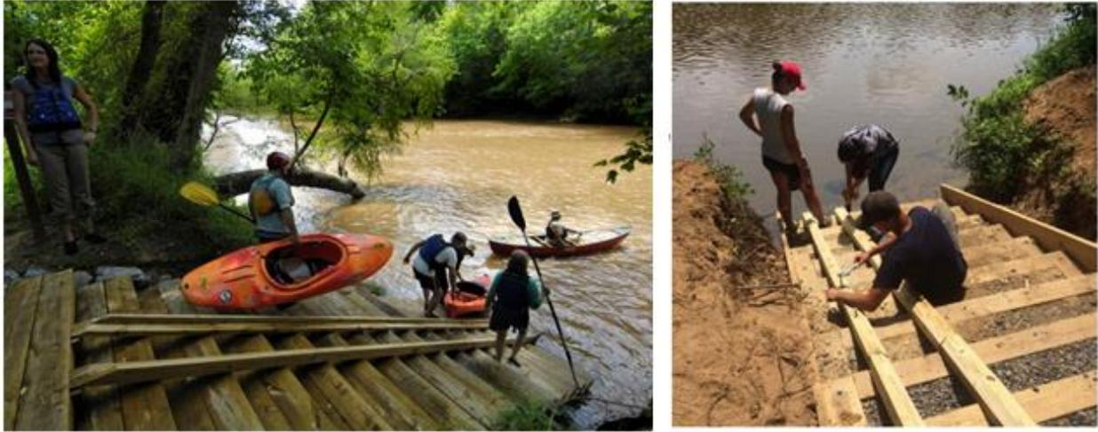
A low impact, “soft” kayak and canoe launch is created to not only make it more convenient and safe to launch, but to reduce the risk of erosion. The existing launches in Windom are mostly mud, so use can increase erosion when people are sliding up and down the bank of the river. There is limited use now, since the launches are not convenient to use.
